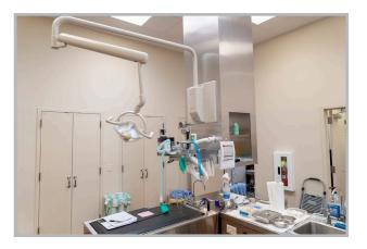
**By mounting anesthesia machines to a wall,** you can provide your staff with a more efficient floor space. There will be less to clean around and fewer items to navigate during patient preparation and surgery.
